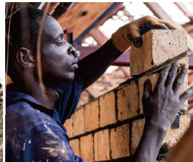
現地で最も汎用性のある焼成レンガを丁寧に積んでいく／ Carefully stacking fired bricks, one of the most versatile materials in the area
