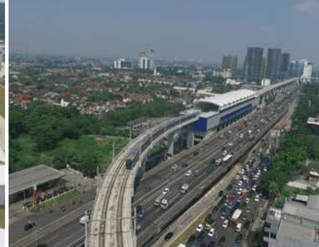
ファトマワティ駅と高速道路を跨ぐ急曲線長大橋／ Long span bridge with small radius curve over toll road near Fatmawati Station
