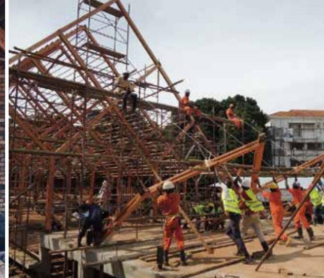
重機を使わず人力で地組したフレームを立ち上げる／ Manually erecting the framework that had been assembled on the ground, without the use of heavy machinery
